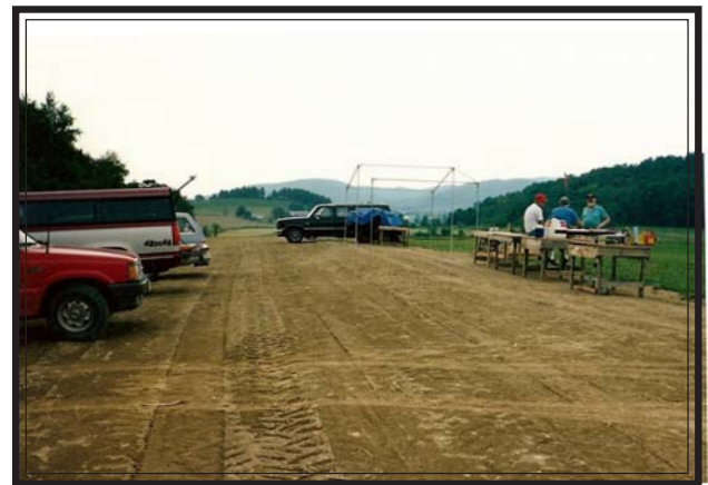
Construction of Pit area. Meerworth field Circa 1990
